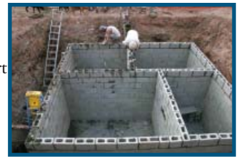
Constructing Tank Walls
